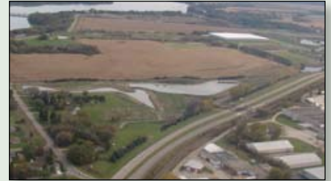
Aerial view of the South Industrial Park Improvement Project on the southwest side of Albert Lea Lake.
