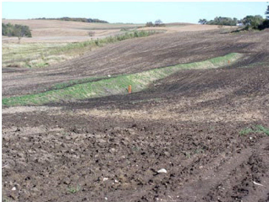
Figure 1. A Water and Sediment Control Basin (Photograph Credit: Swift Soil and Water Conservation District).
